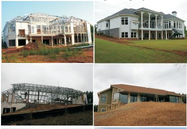
This 9000 sq.ft. Home was built in Conyers, Georgia. Large spans, concrete covered decks and ICF exterior walls set this apart from the rest. It's architecture is Mediterranean. It is magnificent! Steel floor and roof trusses were included as well as interior walls.
